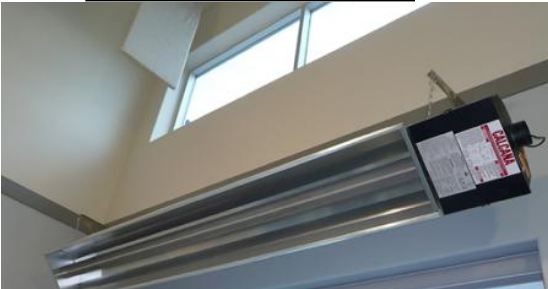
Calcana Infrared Heaters are a good choice for heating sections of warehouses and shops
